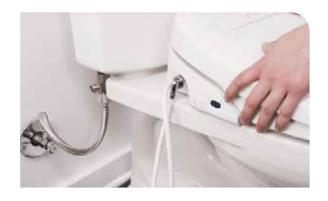
Connect the bidet hose to the bidet, silde the bidet onto the mounting plate
